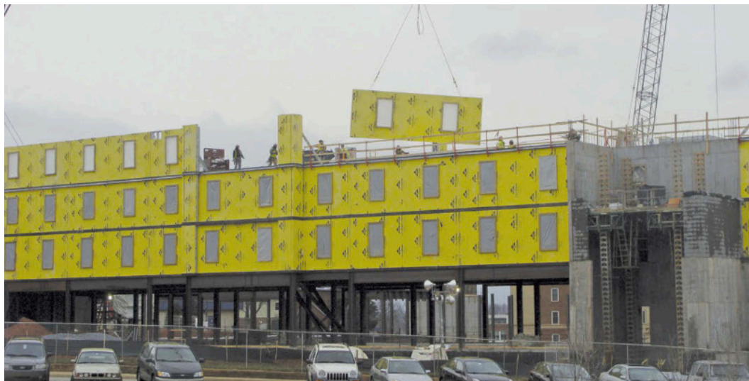
A building constructed by prefabricated panels (Fig. 23)
