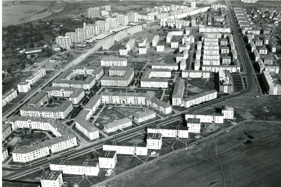
The town of Onesti in Soviet Romania was built entirely from the ground up with prefabricated panels and concrete castings (Fig. 6)
