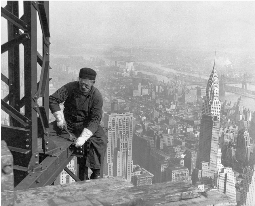
A construction worker tightening steel beams on the Empire State Building of New York City (Fig. 5)
