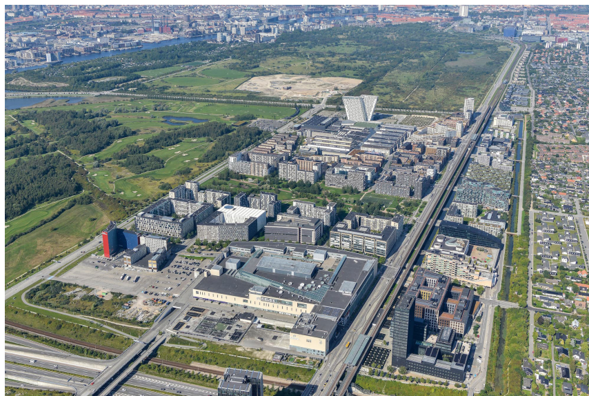
Aerial view of the Ørestad neighborhood (Fig. 37)
