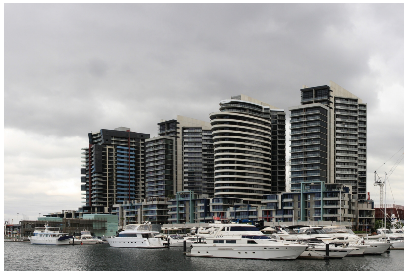
Docklands area, Melbourne Australia (Fig. 20)
