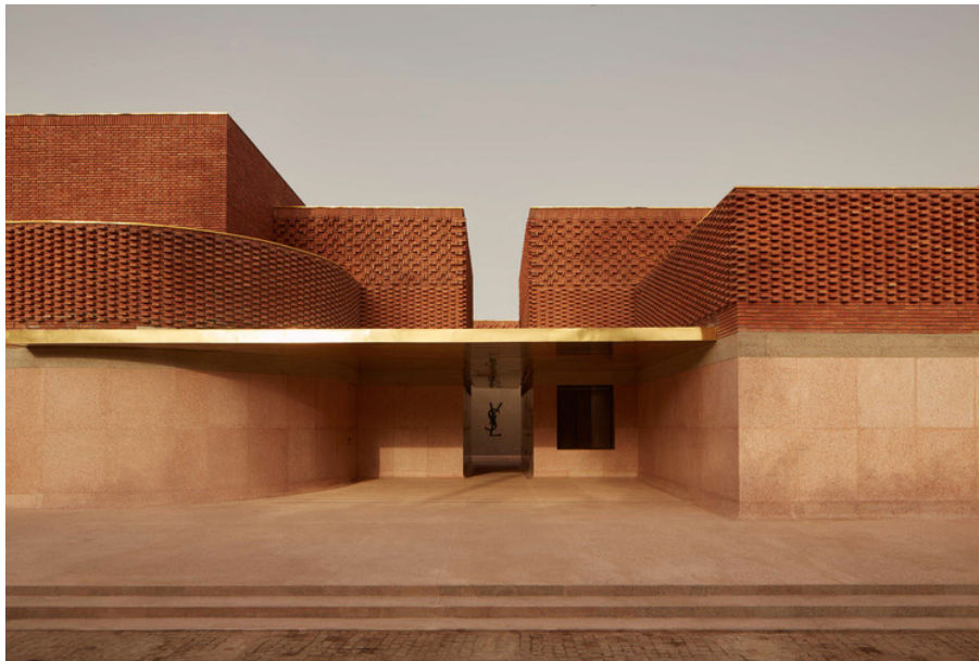
The Yves Saint Laurent museum in Marrakesh, Morocco is heralded as a pristine example of utilizing traditional building techniques in new urban architecture (Fig. 43)
