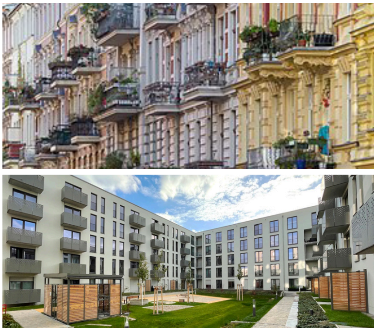
Two modes of housing in the German capital of Berlin – early 20th century brick houses in Bergmannkiez and newly built aluminum and glass houses in the suburb of Adlershof (Fig. 35, Fig. 36)
