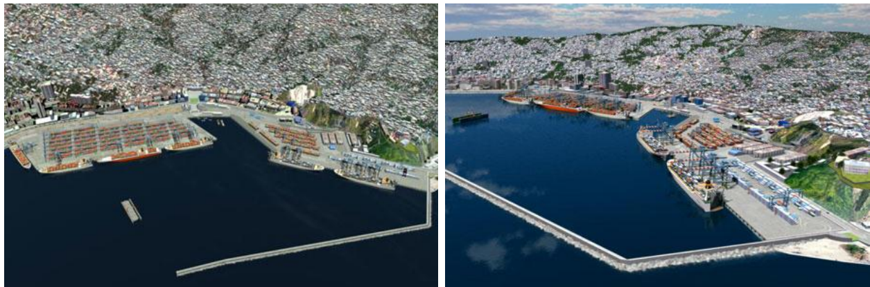
Figure 6 & 7: Images of the terminal II project, the western extension of the Prat Quay (Sources: Valparaiso Port, new challenges of an old port n.d.).
